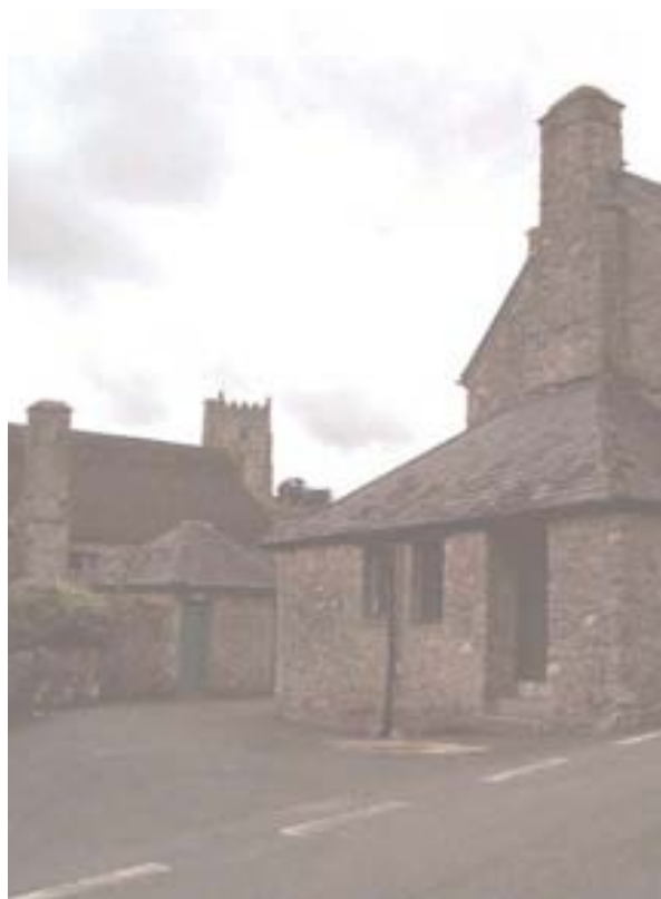
Three outstanding buildings, physically separated but seen viewed as a group
