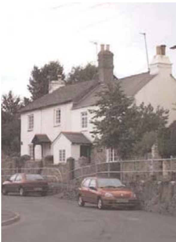
Unlisted buildings can add a great deal to the character of the street scene
