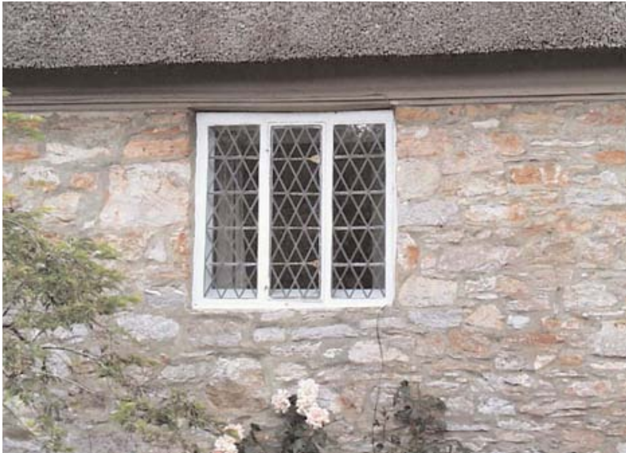
Historically, Church Cottages would've been rendered and/or limewashed. This view, however, illustrates the archetypal building materials of Abbotskerswell
